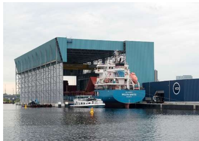
Sheltered terminal, the Netherlands, Figure [www.portofamsterdam.com]
