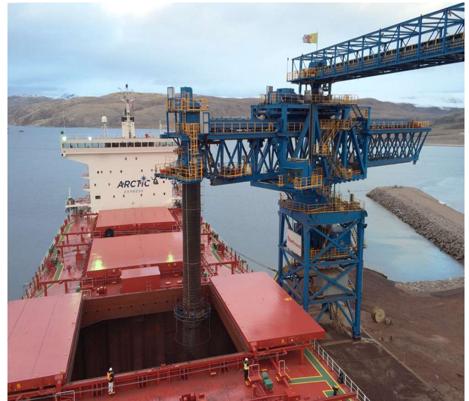
Project: Baffinland Iron Ore Corporation Milne Inlet - Nunavut Canada 2 x SL 3500 tph iron ore, supplied by FAM Beumer Group
