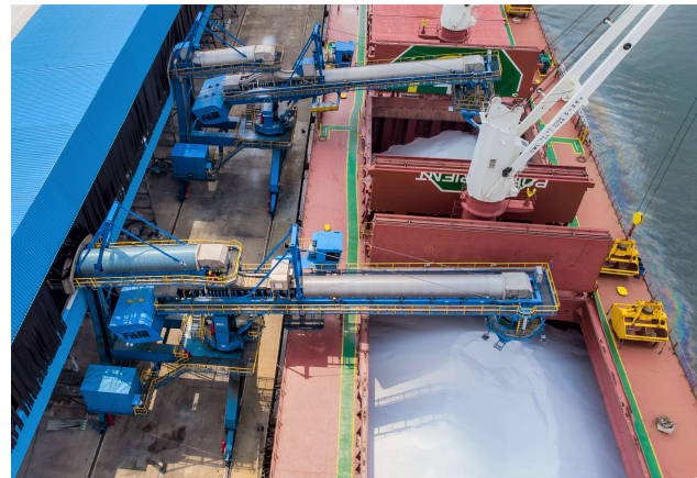
Project: Onne Port, Nigeria SL 990 t/h for urea, FAM Beumer Group
