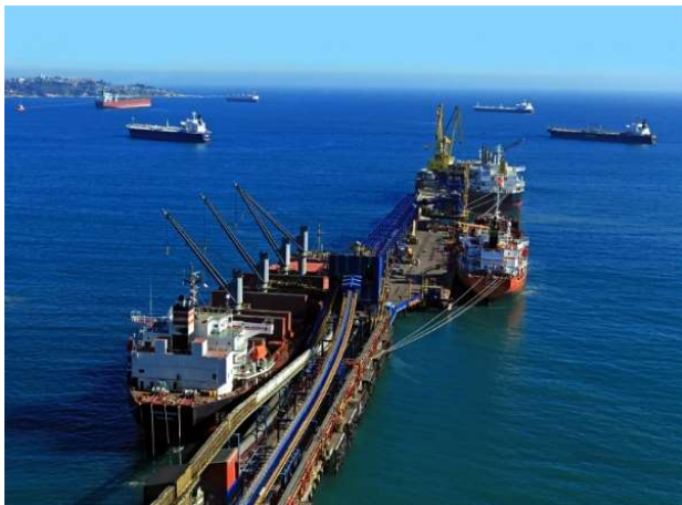
Project: Puerto Ventanas, Chile, pipe conveyors supply by Beumer Group Figure: [www.mundomaritimo.cl]
